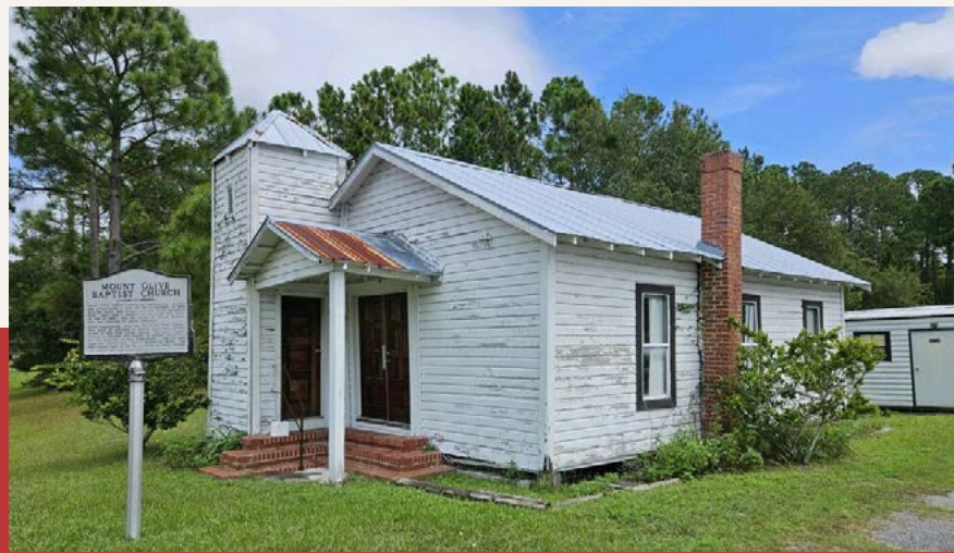
Mount Olive Missionary Baptist Church in Nassau County was listed on the National Register of Historic Places in 1998. The c.1920 frame vernacular church is associated with a congregation that dates to the site in 1870. This church is connected with African-Seminole history and tells the story of African American life in Nassau County. Credit: Tom Keenan
