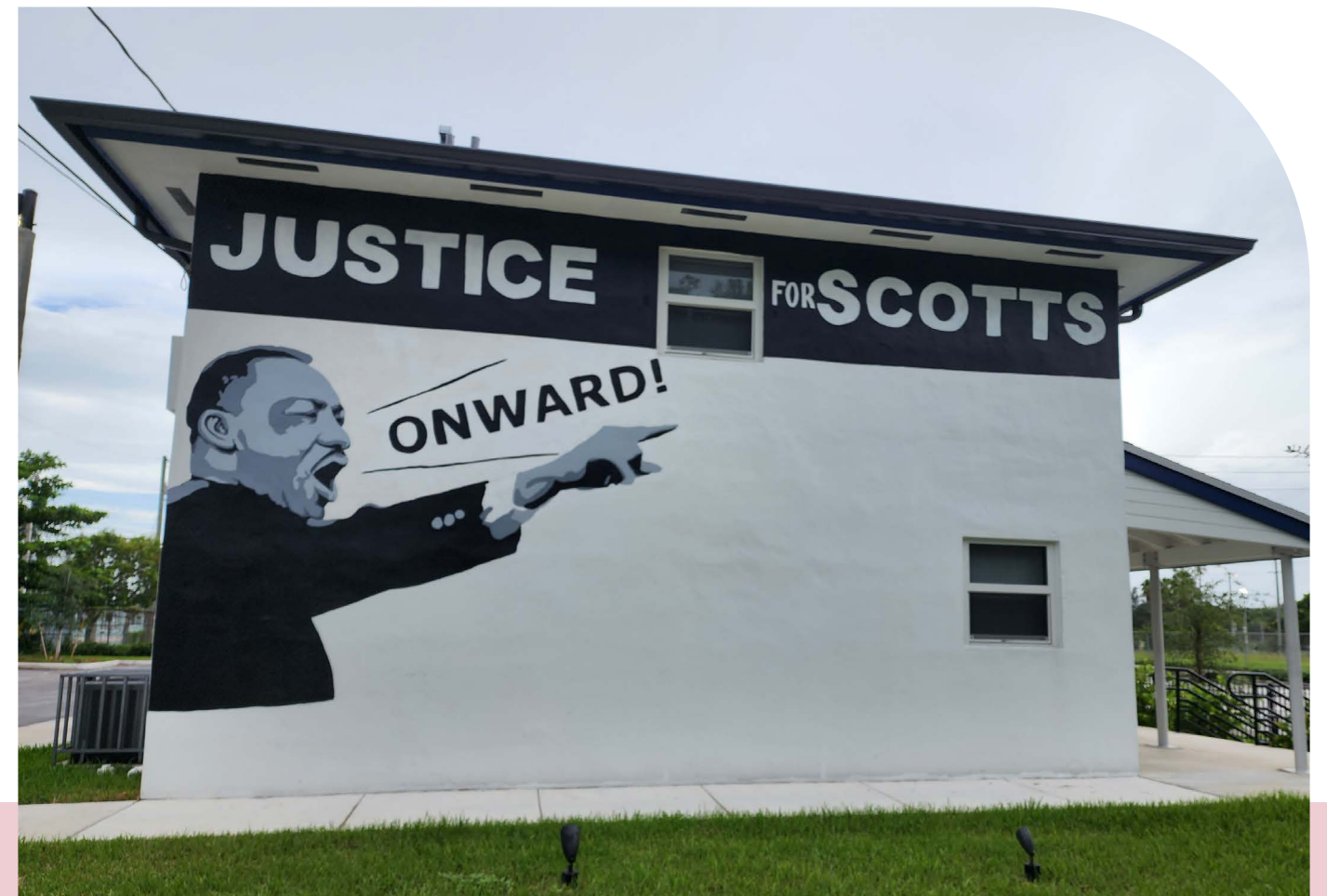
The James E. Scott Homes building in Miami was restored by the Miami-Dade County Public Housing & Community Development department for reuse as housing units. Credit: Sarah Cody-Adelman
