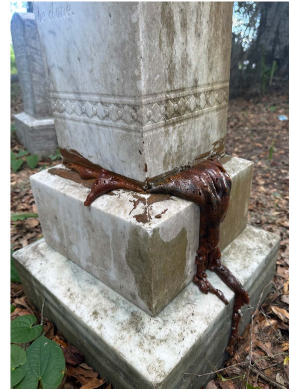
It is best to leave more advanced headstone repair to professionals. The use of incorrect materials can lead to situations such as this epoxy mess on a historic headstone in Ocala. Credit: Adrienne Burke
