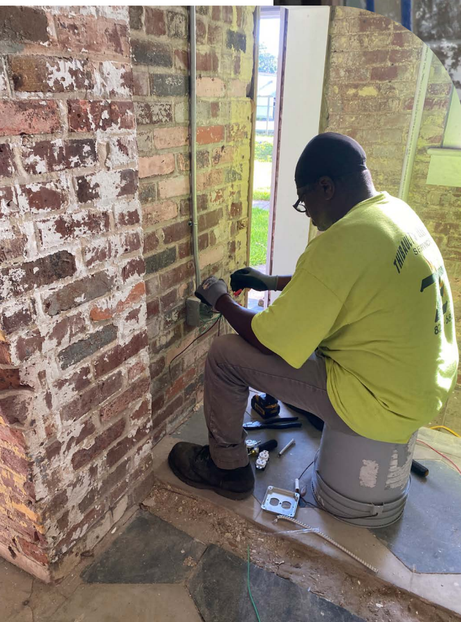
An electrician works on a historic building. Credit: Jennifer Wolfe
