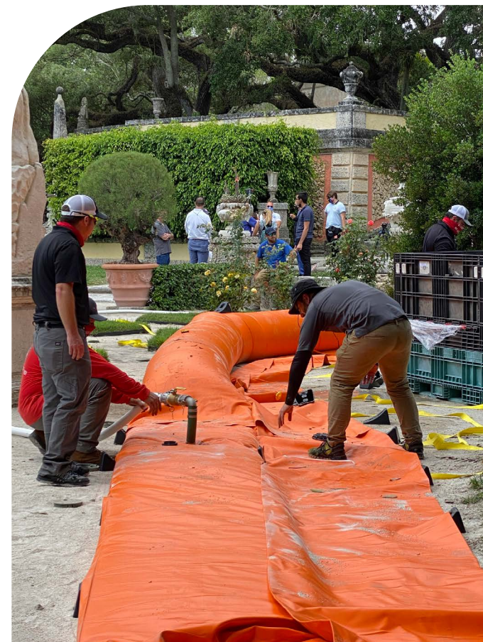
Staff at Vizcaya in Miami do a test deployment on a temporary storm protection measure called a Tiger Dam. It is important to test any storm protection measures in advance to ensure they will be ready for an event. Credit: Adrienne Burke
